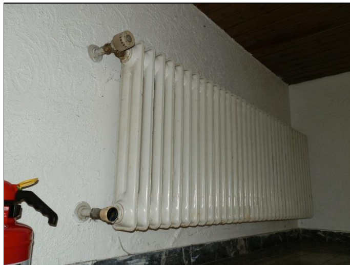
Altes Danfoss-Thermostatventil
